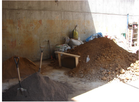
Fig.8 Material tierra y arena
